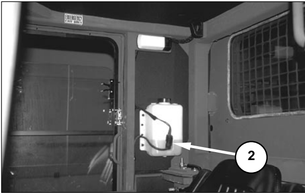
Operator's Compartment, Right Rear Corner. (2) Washer motor.
